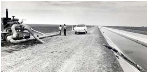
A crew pumps selenium-laden water out of the concrete-lined San Luis Drain into a field near Tranquility, California, in the 1980s as part of a previous cleanup project for selenium-contaminated farm runoff that poisoned birds at the Kesterson National Wildlife Refuge. (Photo Courtesy The Fresno Bee)
