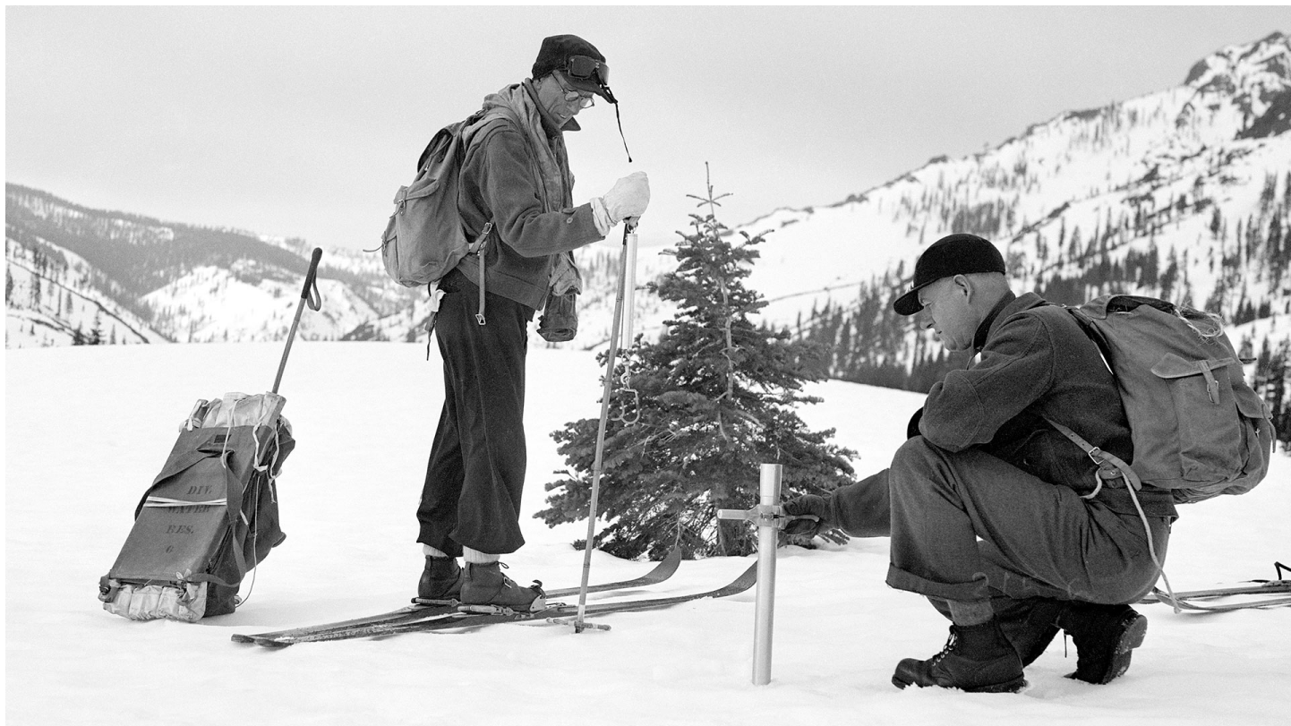
Surveyors using a Mt. Rose snow gauge to measure water content in 1958. Manual surveys are still done the same way. (Calif. Dept. of Water Resources)
